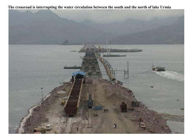
Rebuilding the causaway to a bridge for the passage of cars, trains and ships and guarantee free water circulation in the lake
